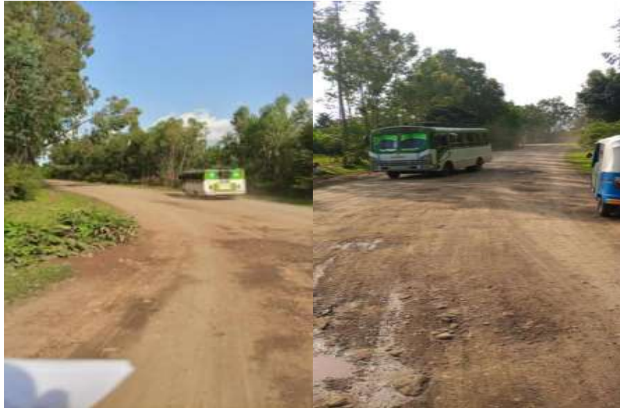
Fig.5: Road condition survey from Areka to Bomebe
